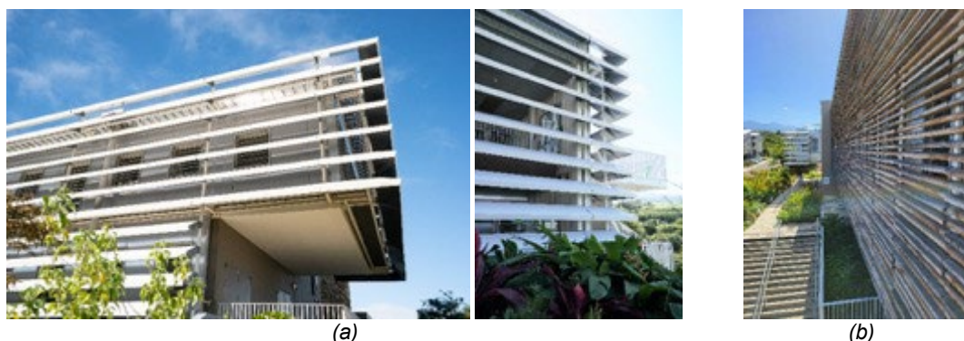
Figure 61: Different solar protection strategies have been set up such as (a) detached horizontal solar shading systems in aluminum and (b) wooden strips
