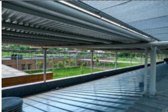
Figure 165: View of the canopy structure. © Emmanuel Museruka – Malaika Media
