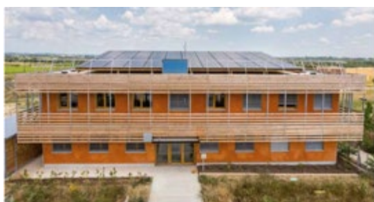
Figure 26 : Exterior view of the Izuba building
