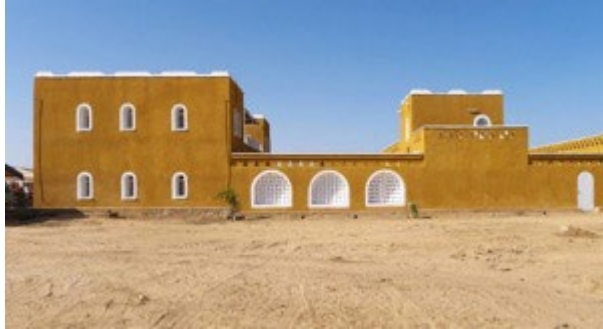
Figure 134 : Exterior view of the 'Maison des Yvelines'.
