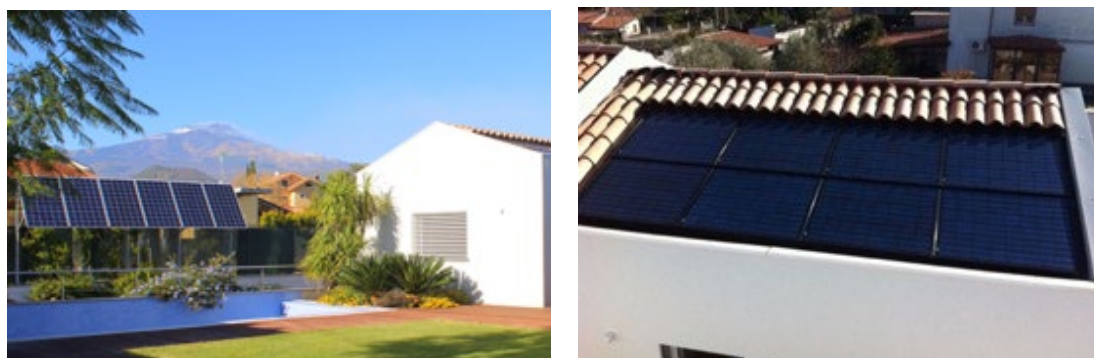
Figure 11: Pictures of photovoltaic System and solar thermal collectors [3]
