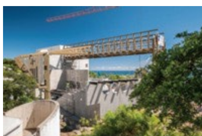
Figure 105 : low pressure shaft under construction
