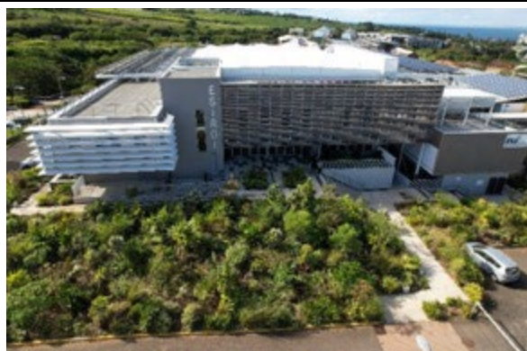
Figure 53 : Exterior view of the eastern façade.
