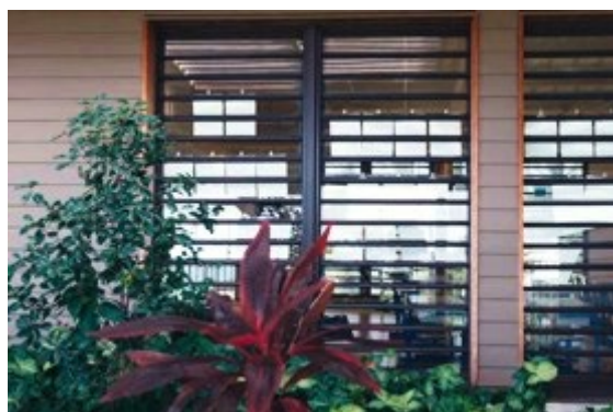
Figure 51 : View of the full-height glass louvers from the exterior corridor
