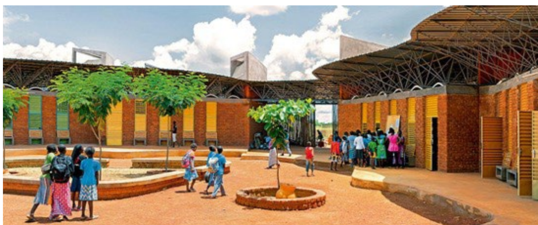
Figure 104: View of the courtyard of the Lycée Schorge © Andrea Maretto for Kéré Architecture.
