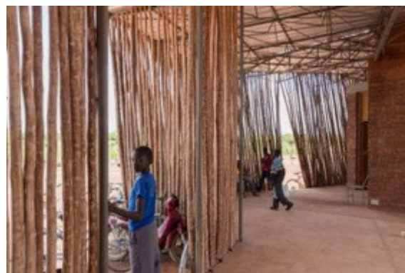
Figure 103 : Wooden screens protect the building from wind, dust and direct solar radiation. © Iwan Baan
