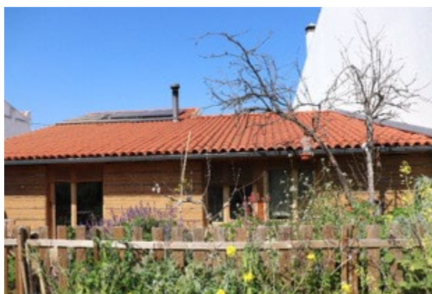
Figure 29 : Exterior view of the main façade in rammed earth and the hanging roof protection made of traditional ceramic tiles.
