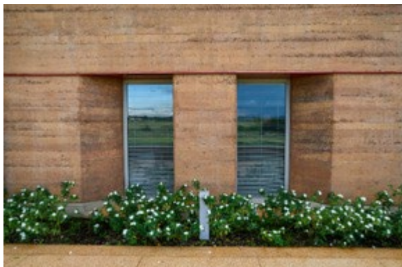
Figure 163: View of the load-bearing walls made of raw earth. © Emmanuel Museruka – Malaika Media
