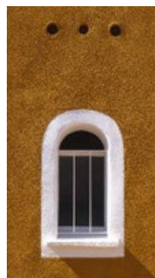
Figure 142 : The different facades present steel windows to allow natural ventilation
