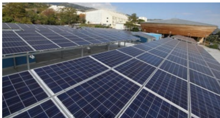
Figure 107: 145 kWp PV panels are installed as shading devices for the cars.
