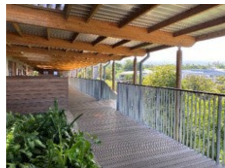
Figure 45: View on the second-floor exterior corridors.
