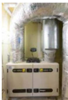
Figure 44 : Double flow mechanical ventilation system
