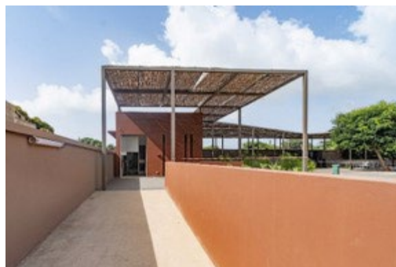
Figure 131: Different solar protection solutions have been set up, such as canopies. ©Daniel Rousselot
