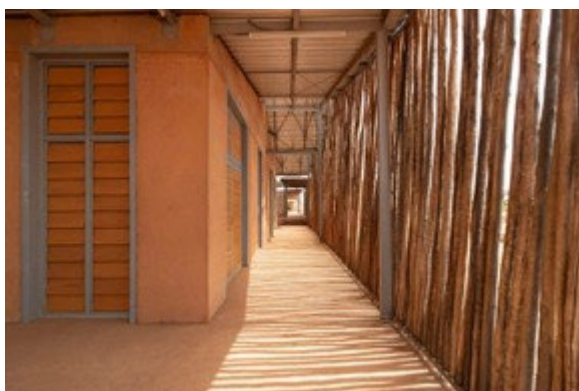
Figure 86: View of a corridor between the classroom and porous skin in eucalyptus wood © Kéré Architecture
