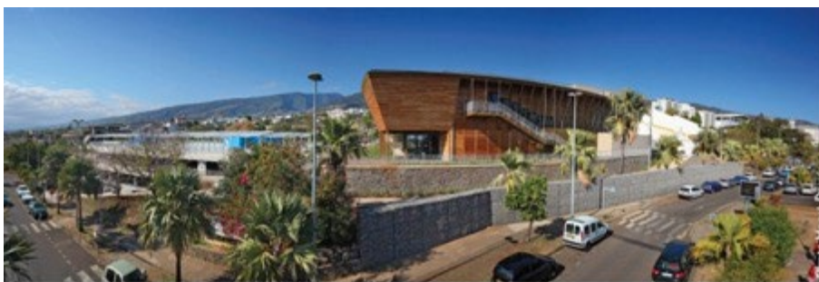
Figure 91 : site integration of the lecture theater
