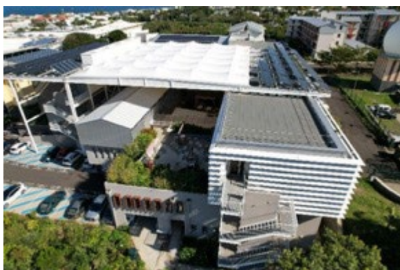
Figure 54 : Exterior view of the western façade.
