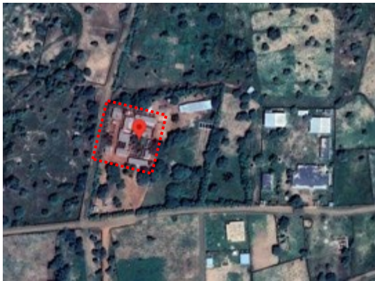
Figure 117: Aerial view of the building.
