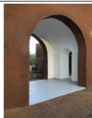
Figure 126: View of the banco walls
