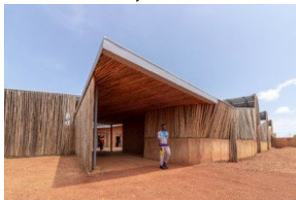
Figure 91: Eucalyptus wood was used to create a porous skin around the building to create a sense of unity with the rest of the campus. © Kéré Architecture
