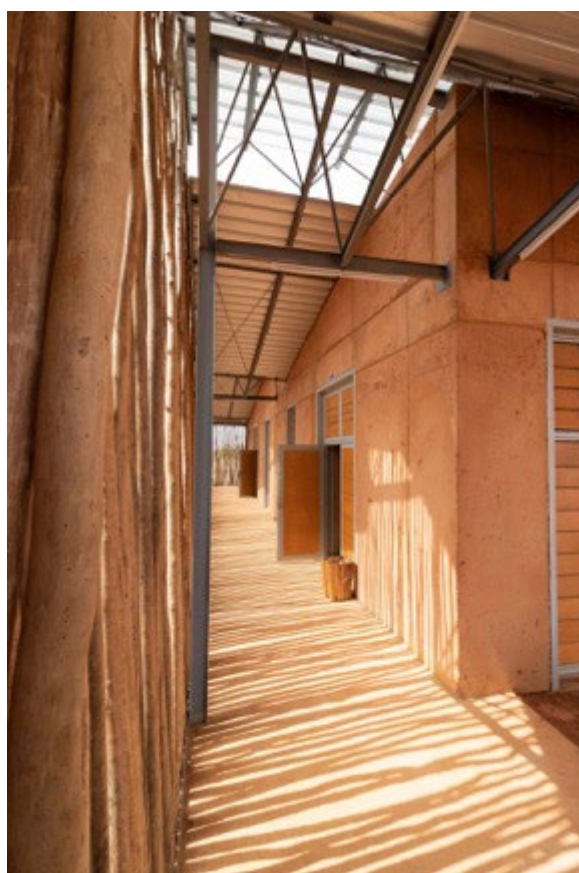
Figure 89: Roof openings allow warm air to be released. © Kéré Architecture
