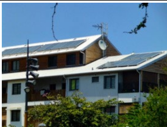
Figure 67 Solar thermal solar panels are installed on the rooftop of the building for the production of hot water
