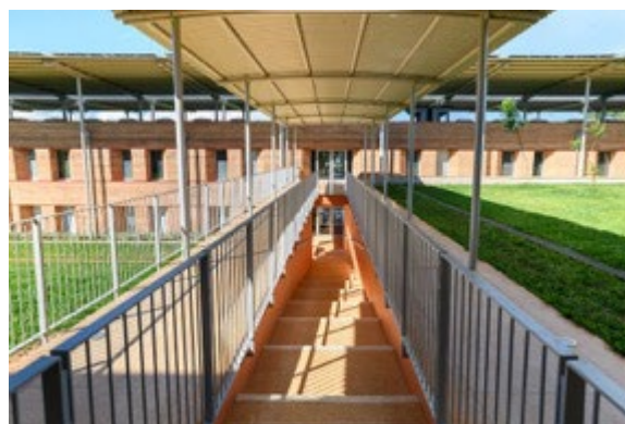
Figure 162 : View of the shaded exterior walkways
