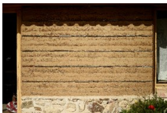
Figure 28: View of the exposed rammed earth wall from the exterior.
