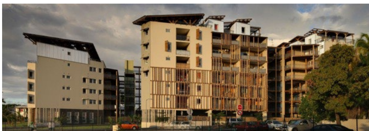
Figure 76: Exterior view of the facades showing the different types of finishing materials used for the exterior walls, i.e., ONDULIT sheet panels and fibre cement siding. © Hervé Douris.
