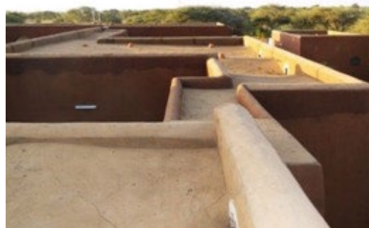
Figure 125: The roof-terrace made of raw clay[1].
