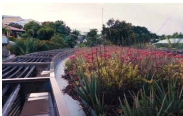
Figure 52 :View of the green roof
