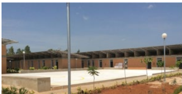
Figure 110 : Exterior view of the CFP Nioro buildings.
