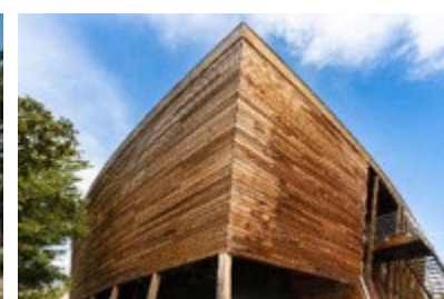
Figure 106 : The external walls are composed of wooden cladding
