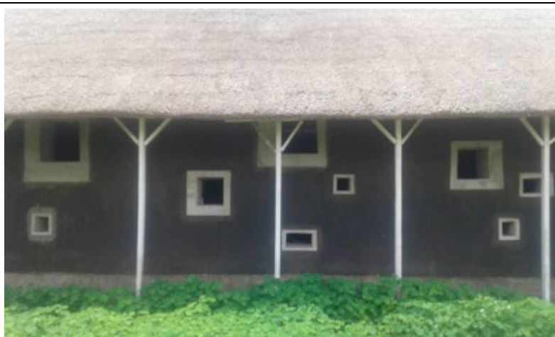
Figure 154 : Exterior view of the East façade of the classroom during the rainy season.
