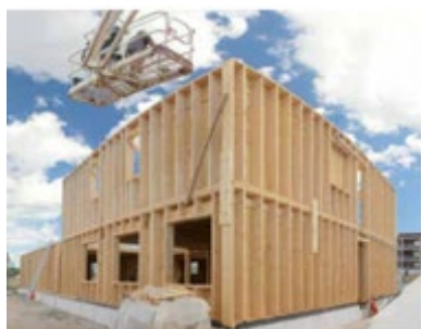
Figure 37: Wood timber structure
