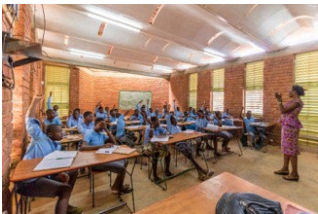
Figure 108: Interior view of a classroom. The undulating ceiling pattern allows to diffuse natural light. © Andrea Maretti for Kéré Architecture
