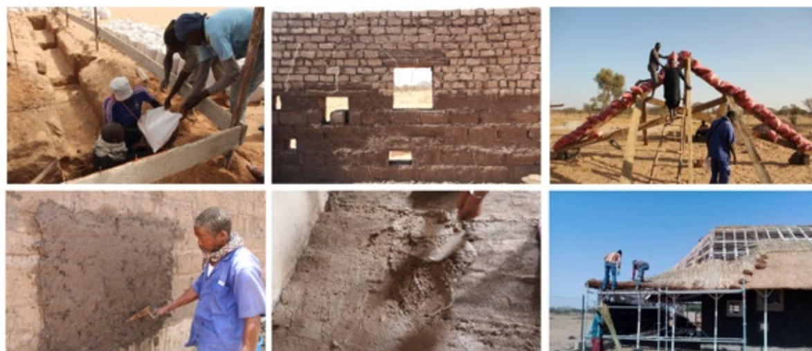
Figure 153 : Construction materials. Top, from left to right: bonded sandbags foundations, mudbrick walls, wooden plank truss. Bottom, from left to right: earth plaster, earth floor and Typha thatched roof.
