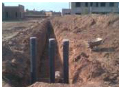
Figure 170: Earth-to-Air Heat Exchanger principle (a) and construction (b) [2]
