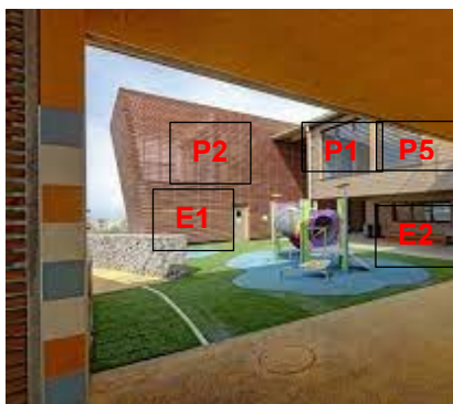
South-East Facade (one can note that sensors P1 and P5 have been placed in classrooms without any solar shadings)
