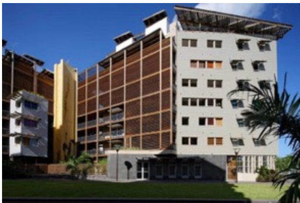
Figure 69 : Optimized solar shading devices, over-roofs and external passageways are architecturally integrated in the Malacca Flores project. (© Hervé DOURIS)
