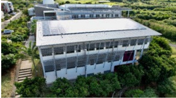
Figure 70 : Southern façade with solar shadings (overhang and wooden strips) [2]
