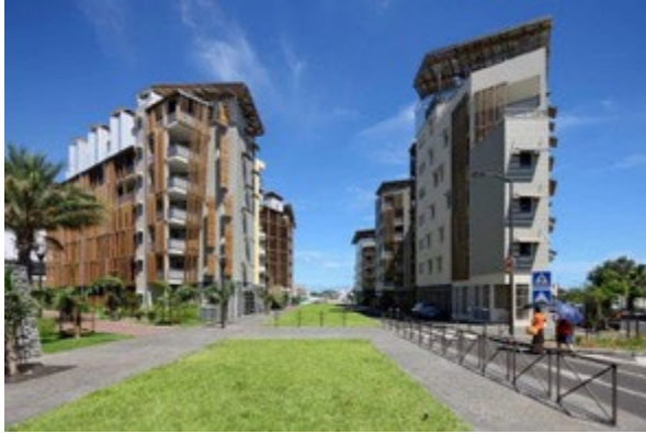
Figure 68 : Exterior view of the Malacca Flores operation and the newly created axis towards the sea. (© Hervé DOURIS)
