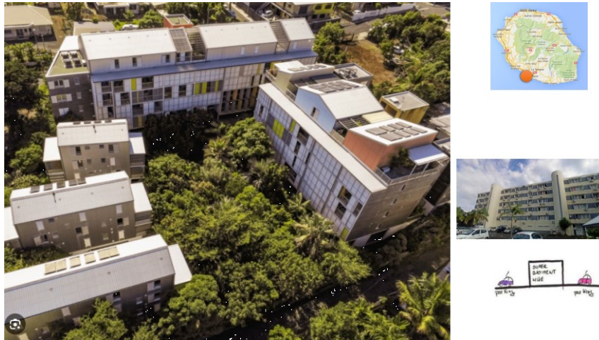
Figure 1 : Native trees has been planted in the heart of the project to cool the outside air. Car parks are located underneath the buildings
