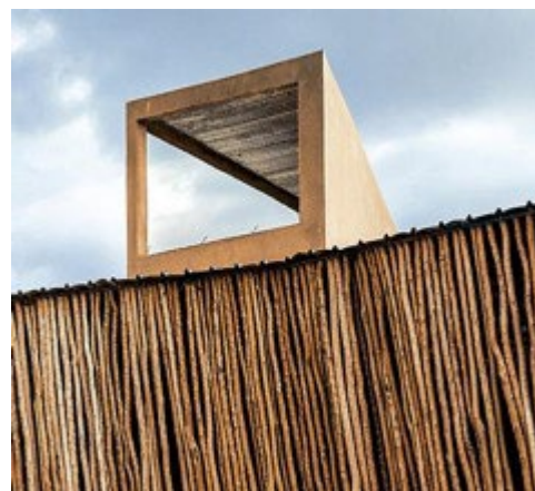
Figure 109 : View of one of the openings at the top of the building ©
