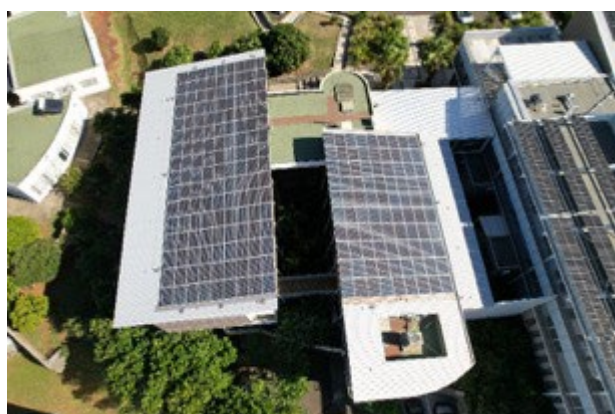
Figure 81 : The 50 kWp BIPV roofs [2]
