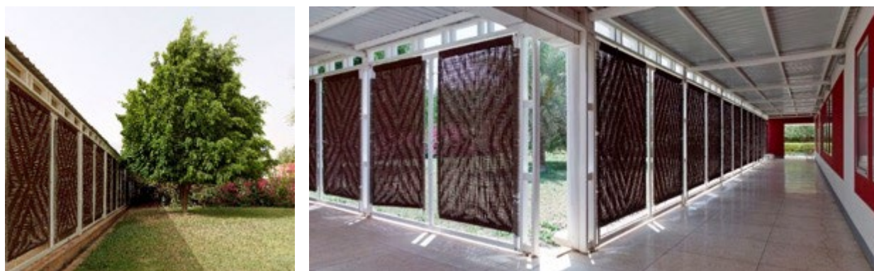
Figure 182: Bamboo sun and dust baffle
