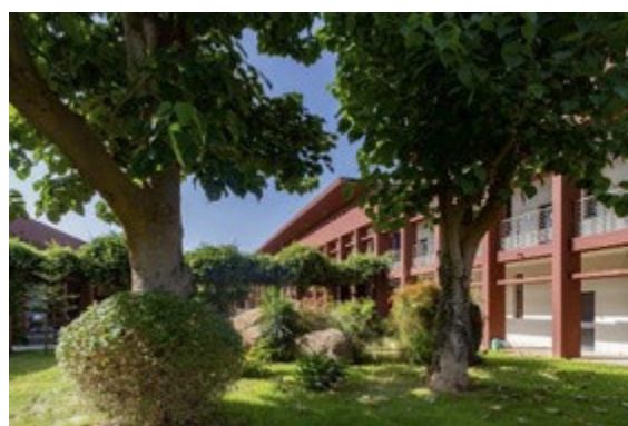
Figure 133: The planted courtyards create a comfortable microclimate around the buildings and also bring conviviality ©Daniel Rousselot
