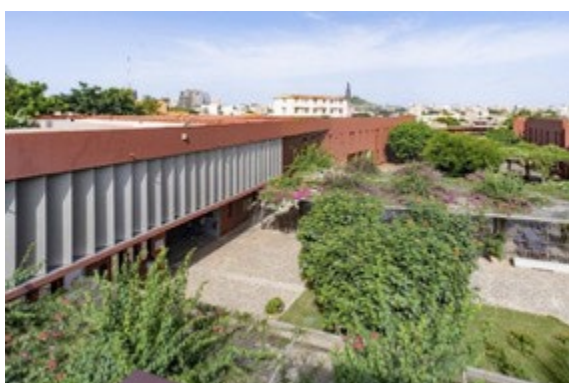
Figure 132 : Solar protection strategies also include vertical blade sunshades and pergolas recovered by climbing plants. ©Daniel Rousselot
