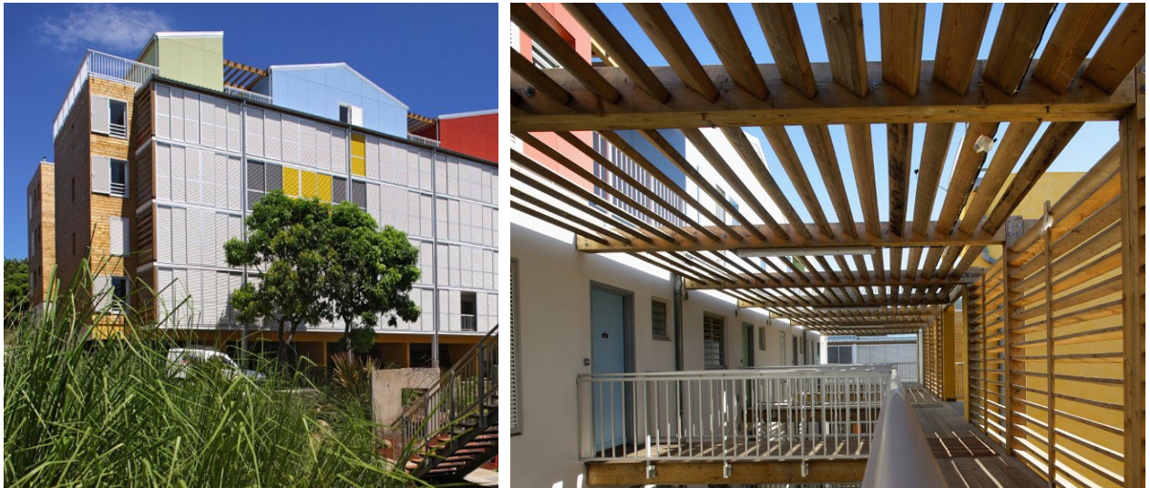
Figure 3 : Light materials (wood or aluminium) are used for solar shadings. Large vertical aluminium louvers have been designed on the veranda side of each apartment to preserve the intimacy of the tenants, to protect the veranda from solar radiation and in the same time to keep the cross natural ventilation by allowing the air to get through the louvers
