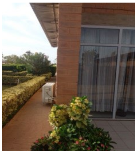
Figure 120: Exterior view of the walls and openings
