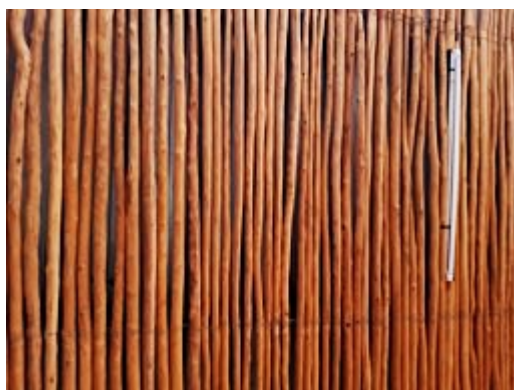
Figure 88 : View of the interior ceilings made of local Eucalyptus wood.
