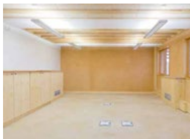
Figure 46 : Lighting of the training room with presence sensors and daylight linked dimming systems
