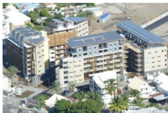
Figure 78 :Aerial view of the PV system and solar thermal panels. (© Hervé Douris)
