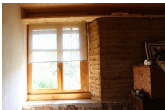
Figure 27: View of the rammed earth wall from the interior.
