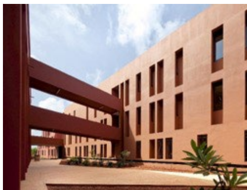
Figure 130: The buildings are connected by exterior corridors. ©Daniel Rousselot
