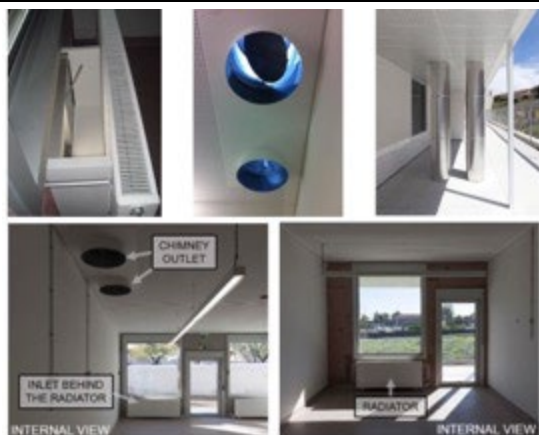
Figure 18 : Elements of the natural ventilation system
