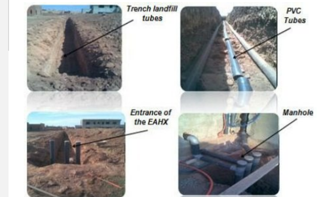
Figure 2: PVC Earth-tubes installation [2]
