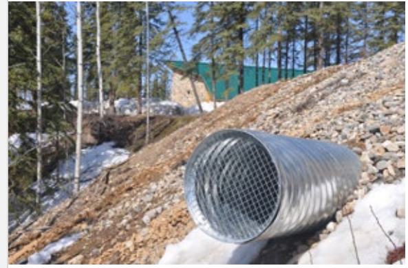
Figure 1: steel earth tube EAHE system air inlet [1]
