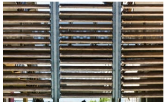
Figure 2: Detail of the fixed shading devices. © Jérôme Balleydier
