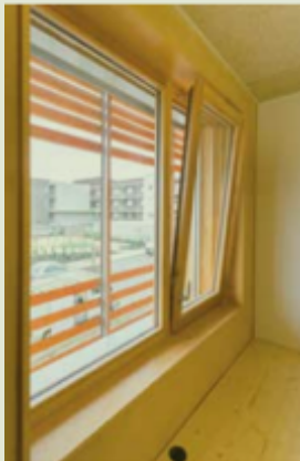
Tilt and turn windows used in Izuba energies building
