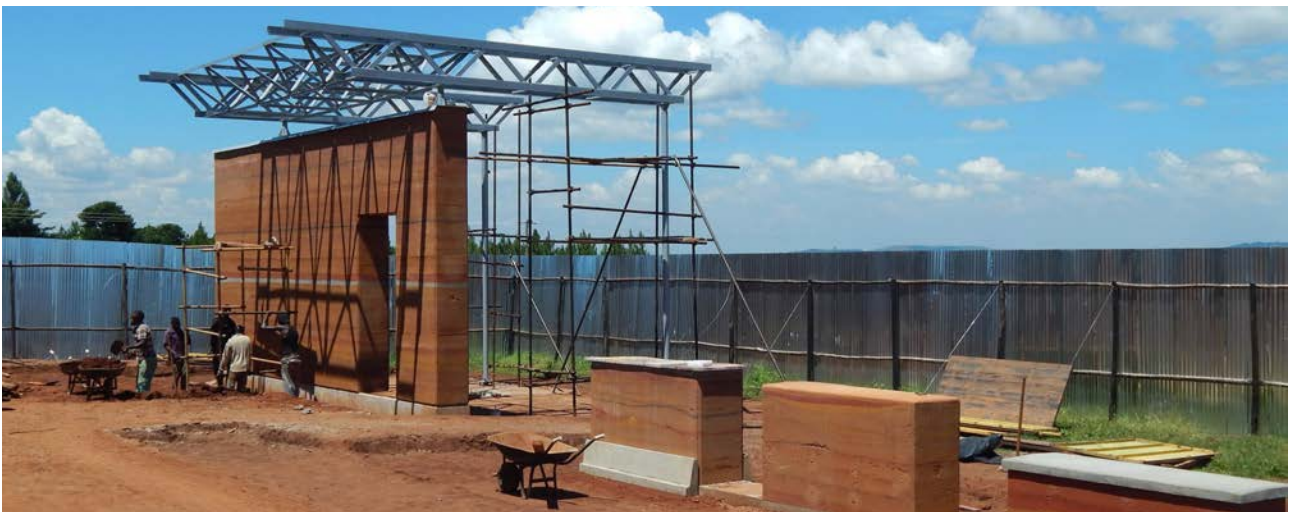
Construction stage © Emergency NGO
