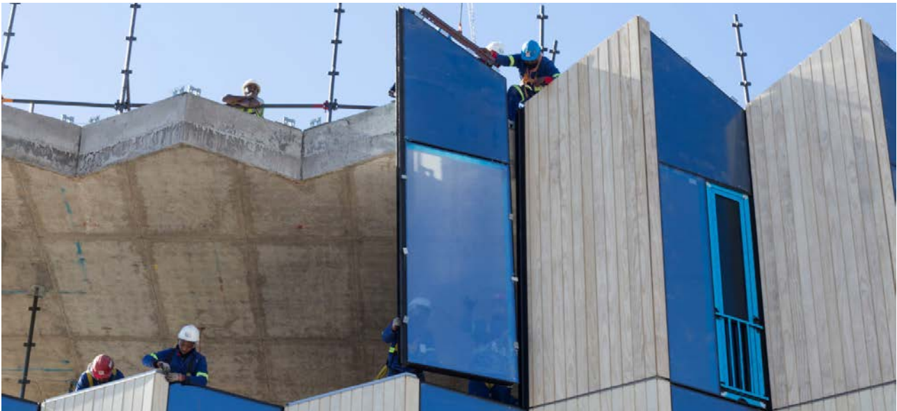
Construction site © Arup
