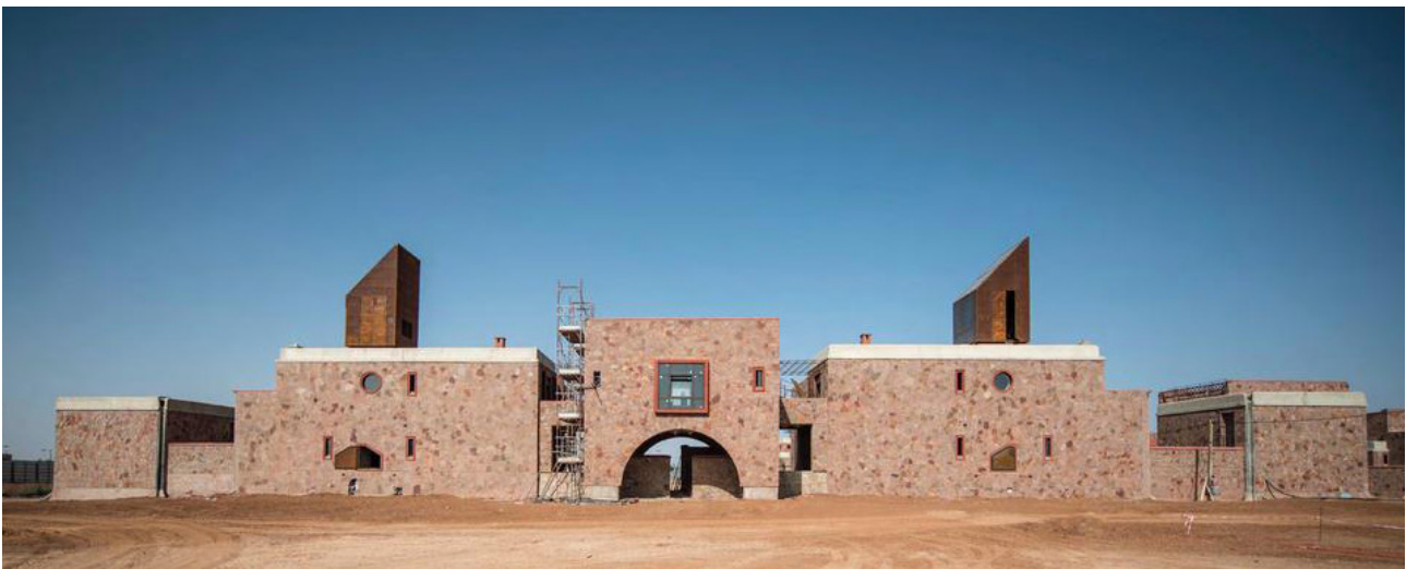
Construction site © Mohammed VI Polytechnic
