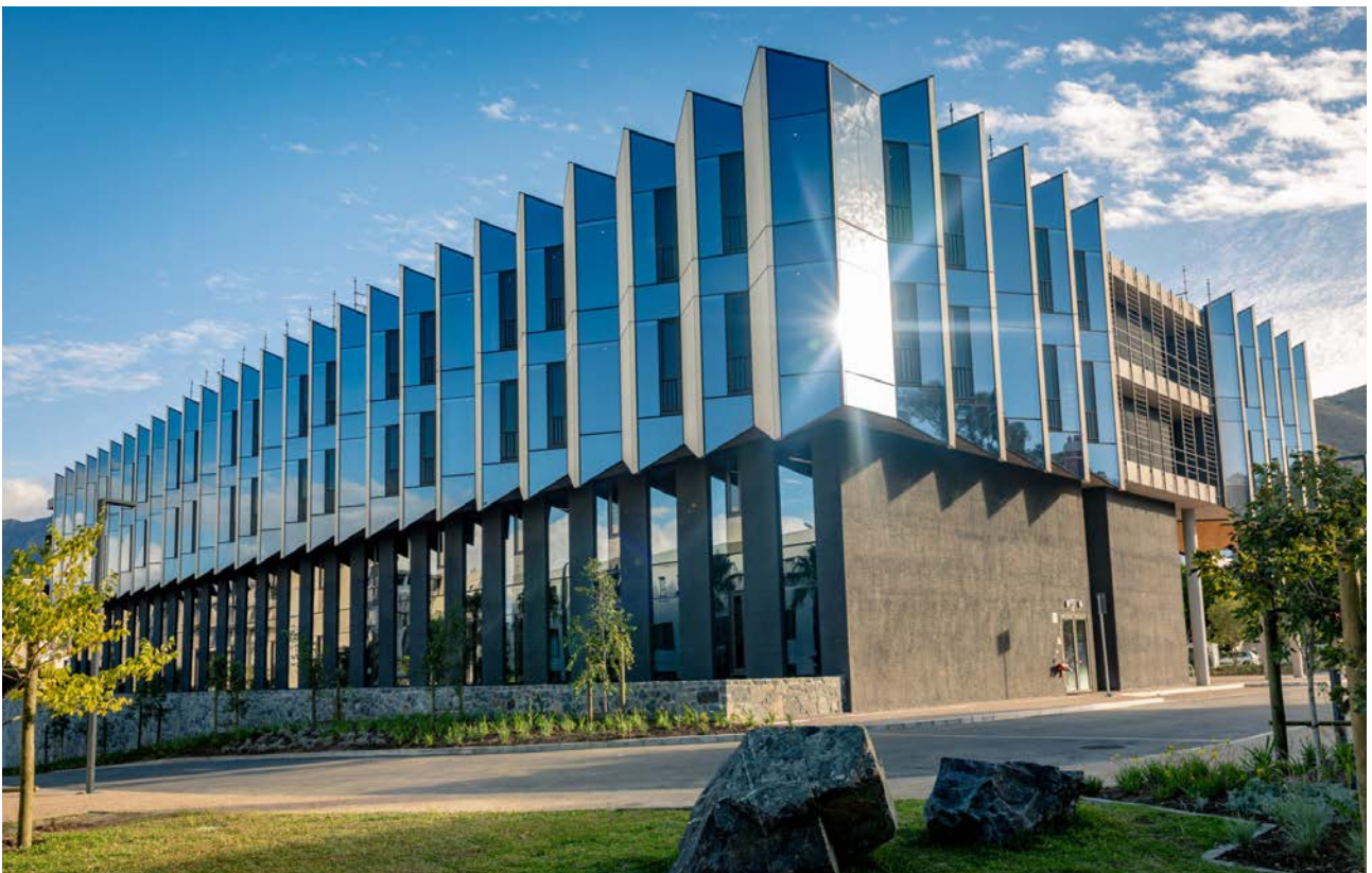
Exterior view © Arup
