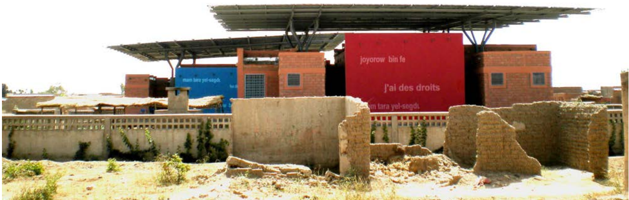
Construction site © FAREstudio
