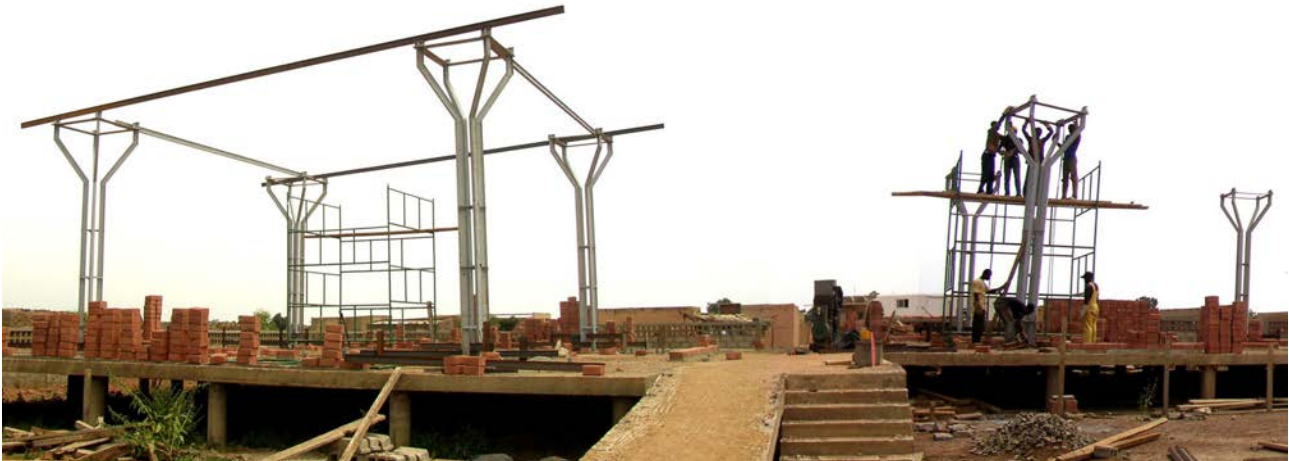
Construction site © FAREstudio
