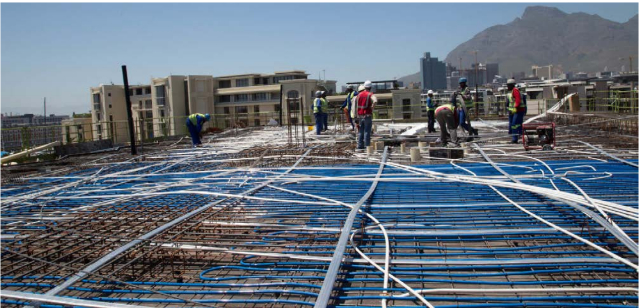
Construction site © Arup
