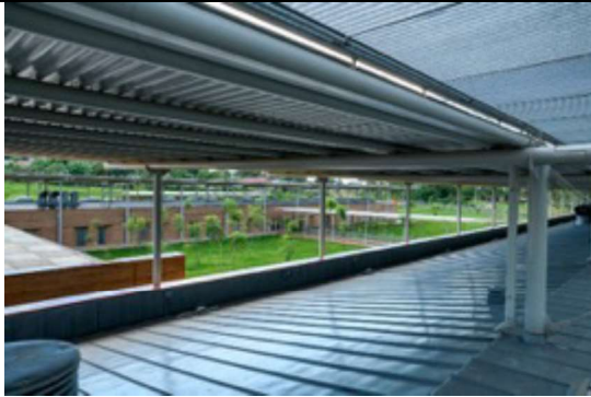
Figure 164: View of the canopy structure. © Emmanuel Museruka – Malaika Media
