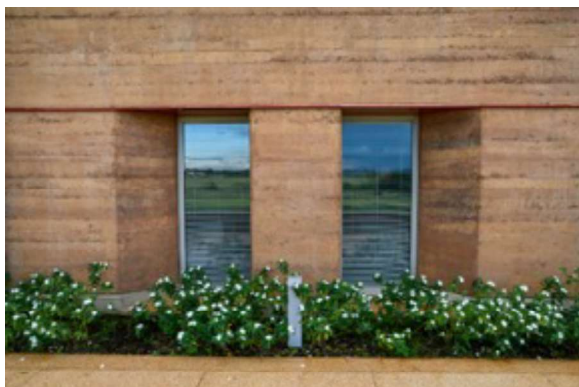
Figure 162: View of the load-bearing walls made of raw earth. © Emmanuel Museruka – Malaika Media
