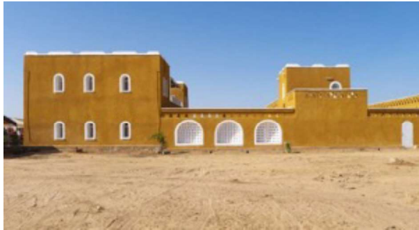
Figure 133 : Exterior view of the 'Maison des Yvelines'.
