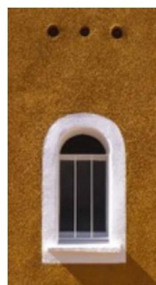
Figure 141 : The different facades present steel windows to allow natural ventilation
