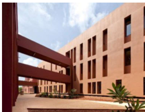
Figure 129: The buildings are connected by exterior corridors. ©Daniel Rousselot
