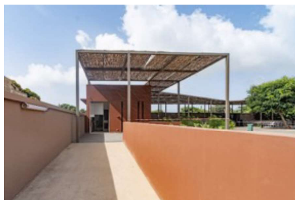
Figure 130: Different solar protection solutions have been set up, such as canopies. ©Daniel Rousselot
