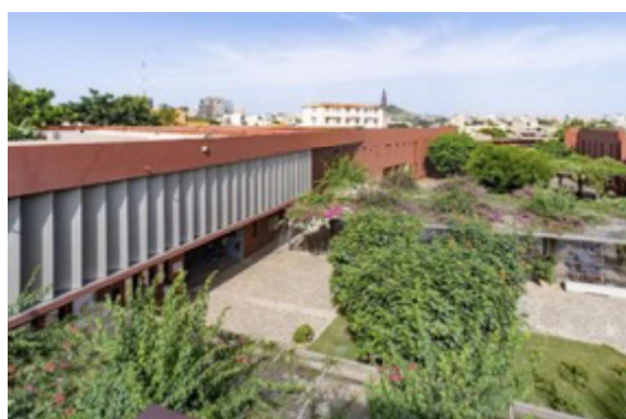
Figure 131 : Solar protection strategies also include vertical blade sunshades and pergolas recovered by climbing plants. ©Daniel Rousselot
