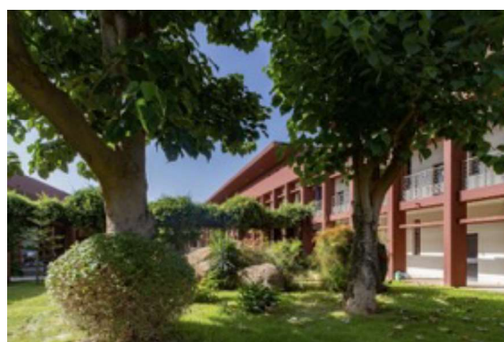
Figure 132: The planted courtyards create a comfortable microclimate around the buildings and also bring conviviality ©Daniel Rousselot
