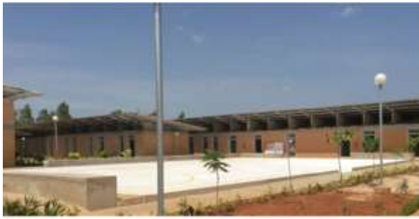
Figure 109 : Exterior view of the CFP Nioro buildings.
