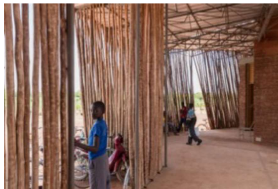
Figure 102 : Wooden screens protect the building from wind, dust and direct solar radiation. © Iwan Baan
