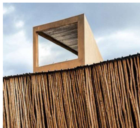
Figure 108 : View of the wind catcher at the top of the building ©
