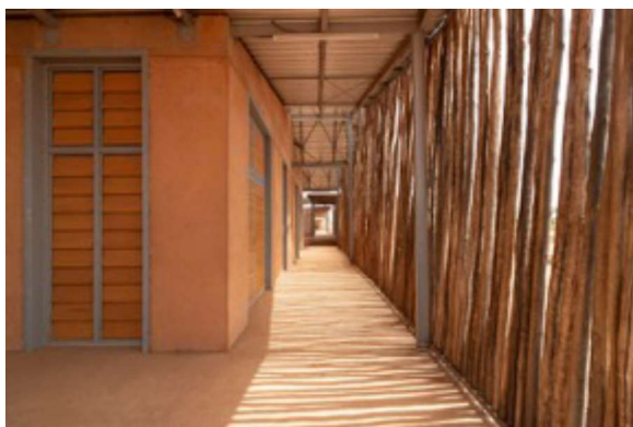
Figure 86: View of a corridor between the classroom and porous skin in eucalyptus wood © Kéré Architecture
