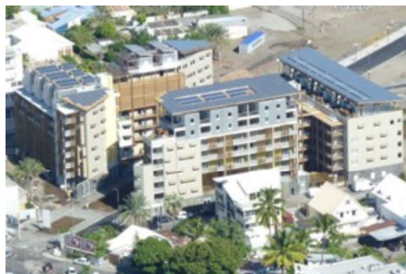
Figure 78 : Aerial view of the PV system and solar thermal panels. (© Hervé Douris)
