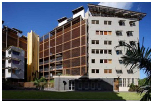
Figure 69 : Optimized solar shading devices, over-roofs and external passageways are architecturally integrated in the Malacca Flores project. (© Hervé DOURIS)
