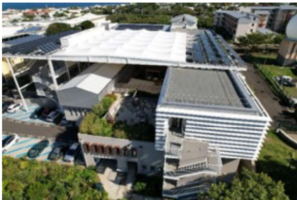
Figure 54 : Exterior view of the western façade.
