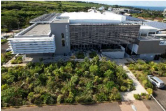
Figure 53 : Exterior view of the eastern façade.
