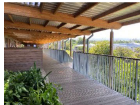
Figure 45: View on the second-floor exterior corridors.
