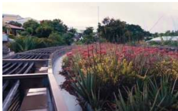
Figure 52 :View of the green roof
