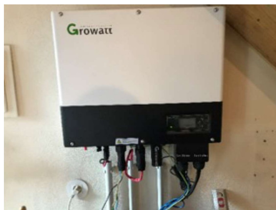
Figure 34 : View of the Growatt Hybrid inverter to PV systems, specially designed for storing current in batteries.
