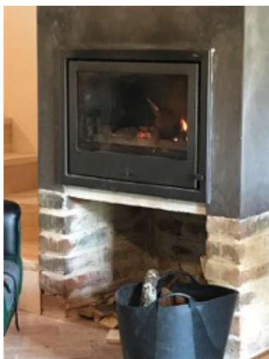
Figure 30 : View of the wood burner.
