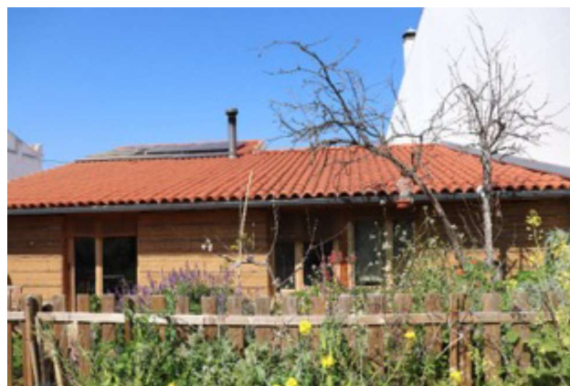
Figure 29 : Exterior view of the main façade in rammed earth and the hanging roof protection made of traditional ceramic tiles.
