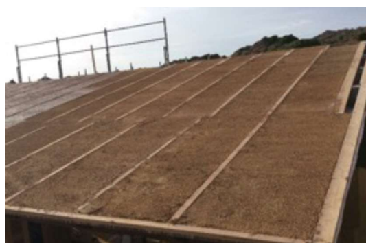
Figure 13 : Construction of the roof: (a) step 1 and (b) step 2.
