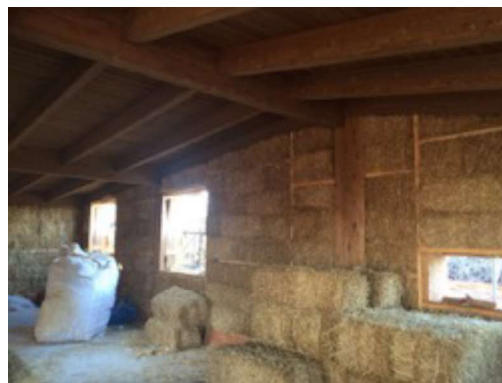
Figure 12: The external walls are highly insulated with straw bales.
