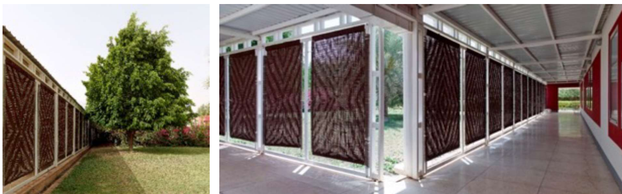
Figure 182: Bamboo sun and dust baffle
