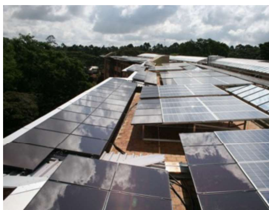
Figure 138: 6000 m 2 of solar panels of 550 kWp are installed on the rooftop of the building [1].
