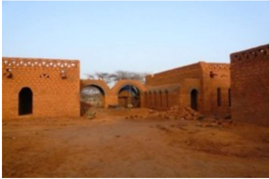
Figure 115: Exterior view of the building « Maison des Energies ». It is a traditional structure in adobe banco.
