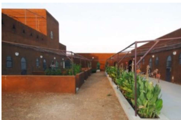
Figure 121: View of the exterior courtyard of the « Maison des Energies » and its garden [1].
