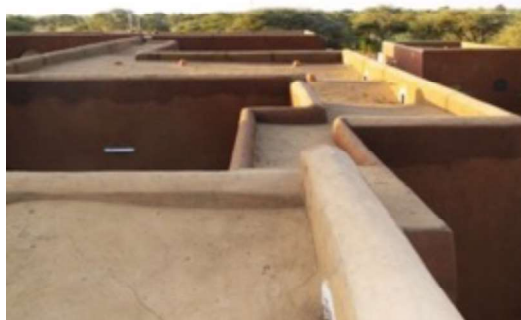
Figure 125: The roof-terrace made of raw clay[1].
