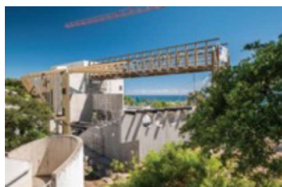
Figure 105 : low pressure shaft under construction
