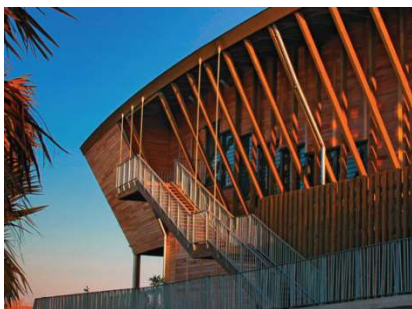
Figure 101 : Solar shadings
