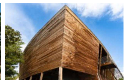
Figure 106 : The external walls are composed of wooden cladding
