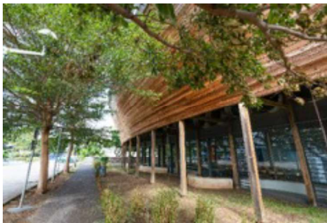
Figure 88: Eastern facade with air inlets and native vegetation
