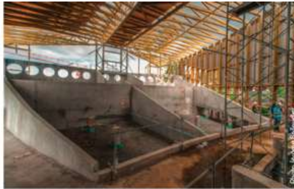
Figure 99 : Construction of the air compartments during the construction stage
