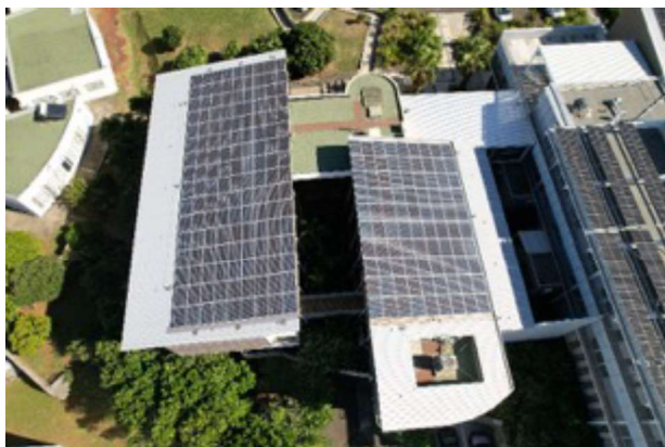
Figure 81 : The 50 kWp BIPV roofs [2]
