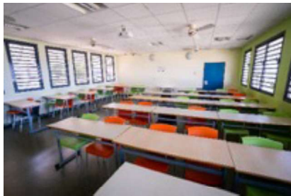
Figure 78 : a typical classroom with large louvers on both sides and efficient ceiling fans [2]
