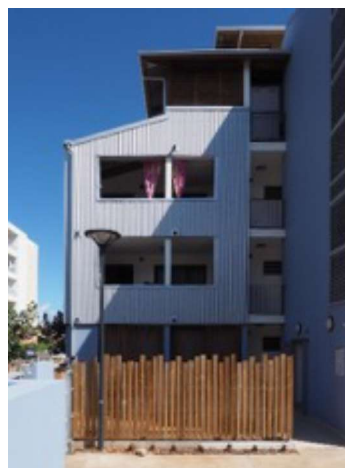
Figure 65: Exterior wall made with the Mauka Brizz system. Photo credits: N. Peyrebonne.
