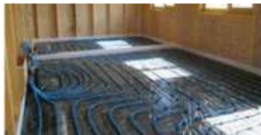
Figure 43: The building is equipped with an under-floor heating/cooling system powered by a ground source heat pump
