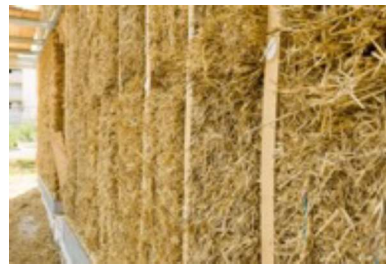
Figure 38: Bunches of straw and wood fiber insulation in exterior walls
