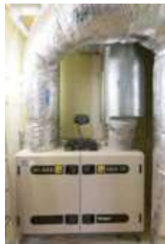
Figure 44 : Double flow mechanical ventilation system
