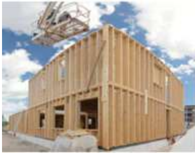
Figure 37: Wood timber structure
