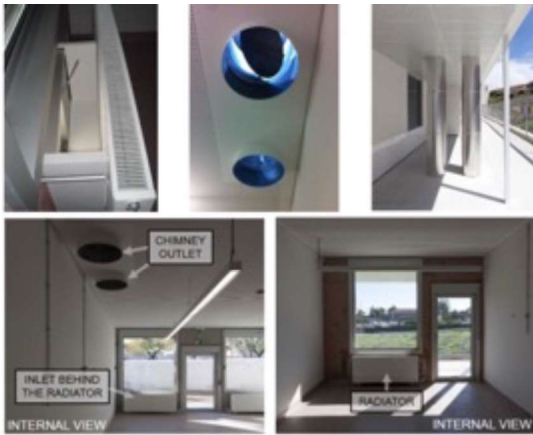
Figure 18 : Elements of the natural ventilation system
