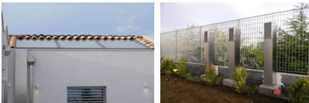
Figure 10: Pictures of installed systems (on the left: thermal solar collectors, on the right: Earth to Air Heat Exchanger) [3]
