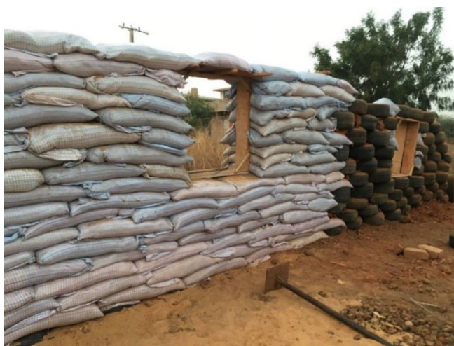
Figure 18: Building a school in Ngekhokh / source: https://www.letsbuildmyschool.org/
