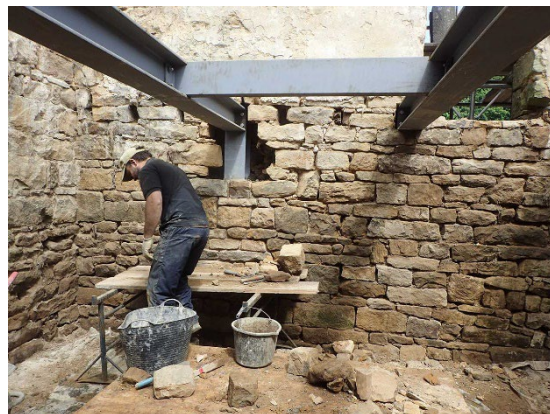
Figure 6: Stone building during construction
