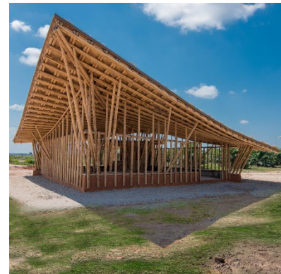
Figure 8: A bamboo construction.
