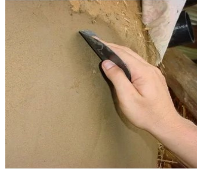
Figure 2: Plastering a wall Photo credit: Travis Toon. Source: https://www.dancingrabbit.org/about-dancing-rabbit-ecovillage/eco-living/building/natural-building/earthen-plaster/
