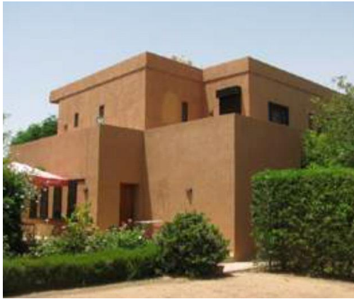
Figure 156: Exterior view of the Dar Amys Villa
