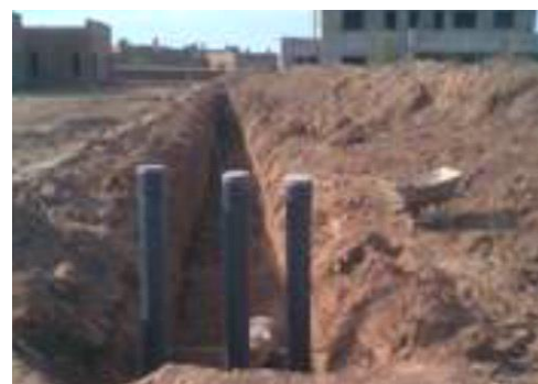
Figure 163: Earth-to-Air Heat Exchanger principle (a) and construction (b) [2]
