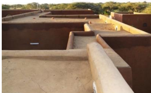
Figure 118: The roof-terrace made of raw clay[1].
