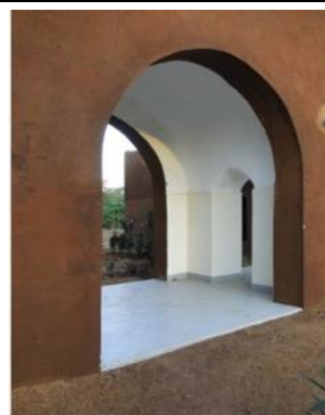
Figure 119: View of the banco walls
