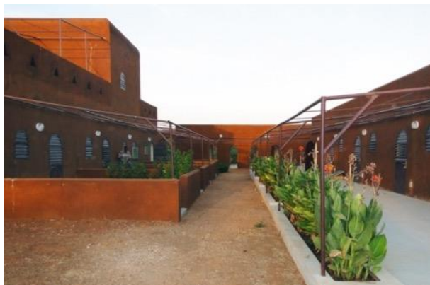
Figure 114: View of the exterior courtyard of the « Maison des Energies » and its garden [1].
