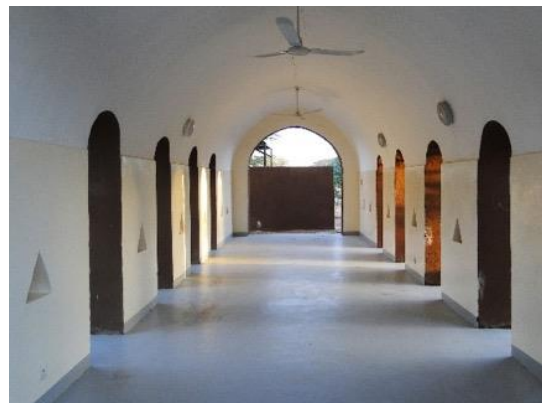
Figure 115: Interior view of the building “Maison des Energies” with the ceiling fans [1].
