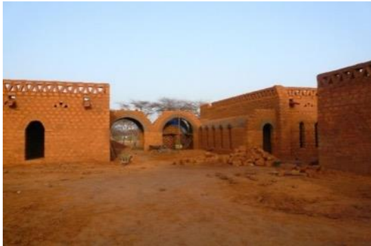
Figure 108: Exterior view of the building « Maison des Energies ». It is a traditional structure in adobe banco.
