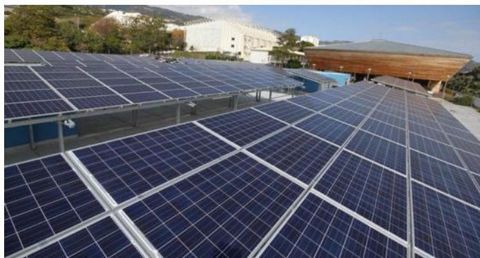
Figure 101: 145 kWp PV panels are installed as shading devices for the cars.
