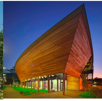
Figure 97 : The external walls are composed with wooden cladding
