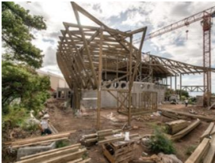
Figure 95 : wooden superstructure
