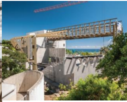
Figure 96 : low pressure shaft under construction
