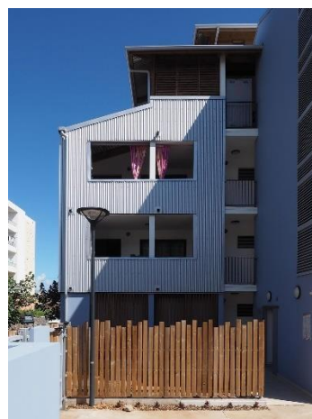
Figure 59: Exterior wall made with the Mauka Brizz system. Photo credits: N. Peyrebbonne.
