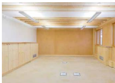
Figure 45 : Lighting of the training room with presence sensors and daylight linked dimming systems
