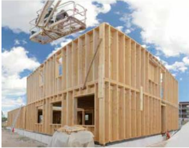
Figure 36: Wood timber structure
