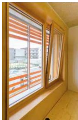
Figure 35: Tilt and turn windows
