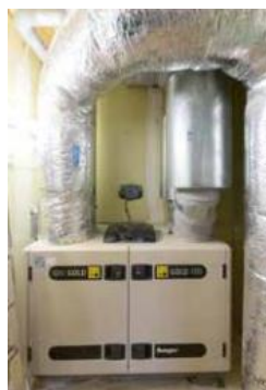
Figure 43 : Double flow mechanical ventilation system
