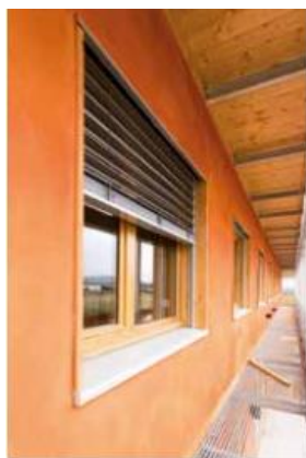
Figure 34: Motor drive external venetian blind. Type: Grinotex from Griesser.
