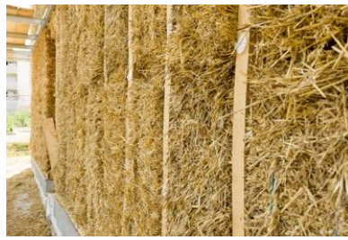
Figure 37 Bunches of straw and wood fiber insulation in exterior walls
