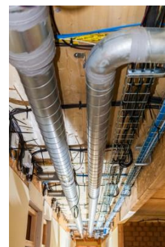
Figure 44 : Air distribution system of the building
