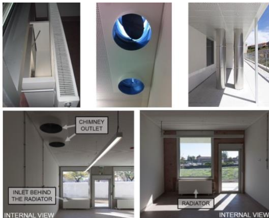
Figure 18 : Elements of the natural ventilation system
